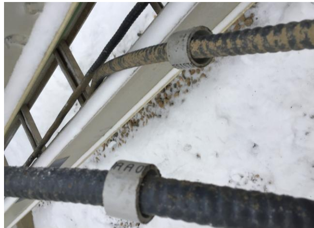
Figure 2 – Removal of Multiple Cables
