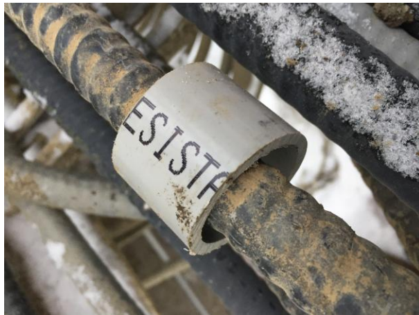
Figure 1 - Installation of "Donut"
