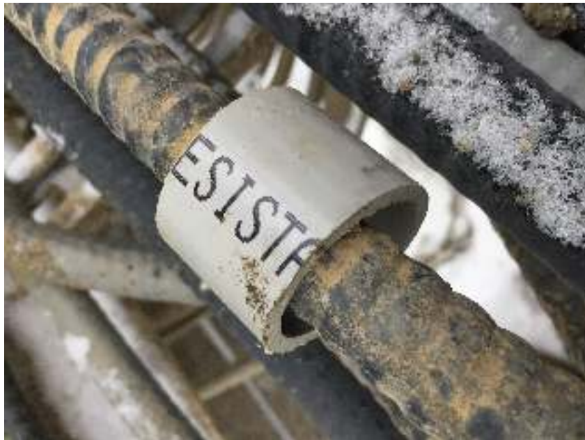
Figure 1 - Installation of "Donut"
