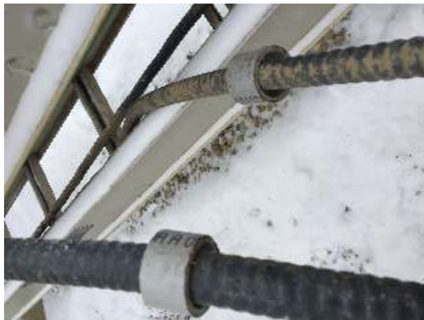
Figure 2 – Removal of Multiple Cables
